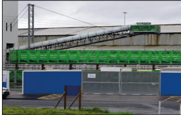
Noise Control Shieldhall Strategic Tunnel, Glasgow
