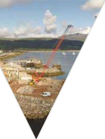
A five-phase construction programme ensured that construction works were carried out with no detriment to live port operations. Detailed traffic management plans enabled progress whilst maintaining an uninterrupted ferry service.
